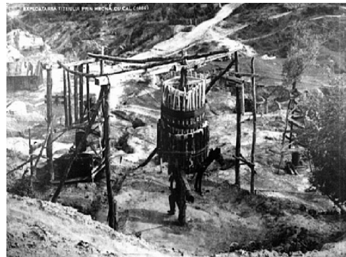
Crude oil extraction
